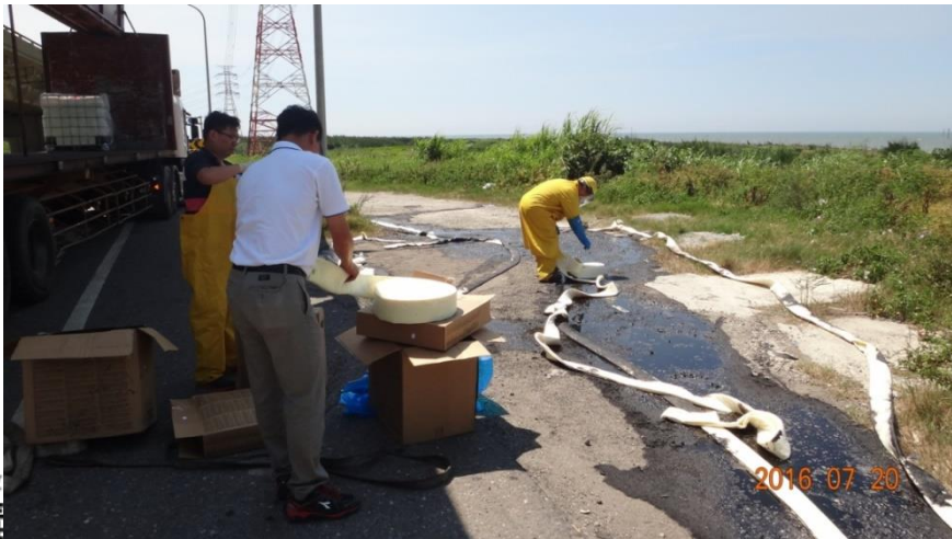
Absorbing sulfuric acid with absorbent cotton
