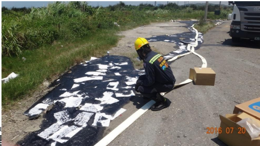
Absorbing sulfuric acid with absorbent cotton
