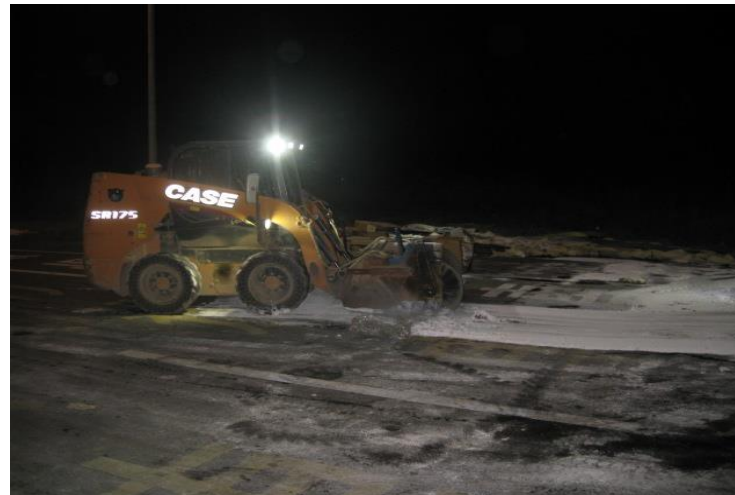
Remove the ground lime
