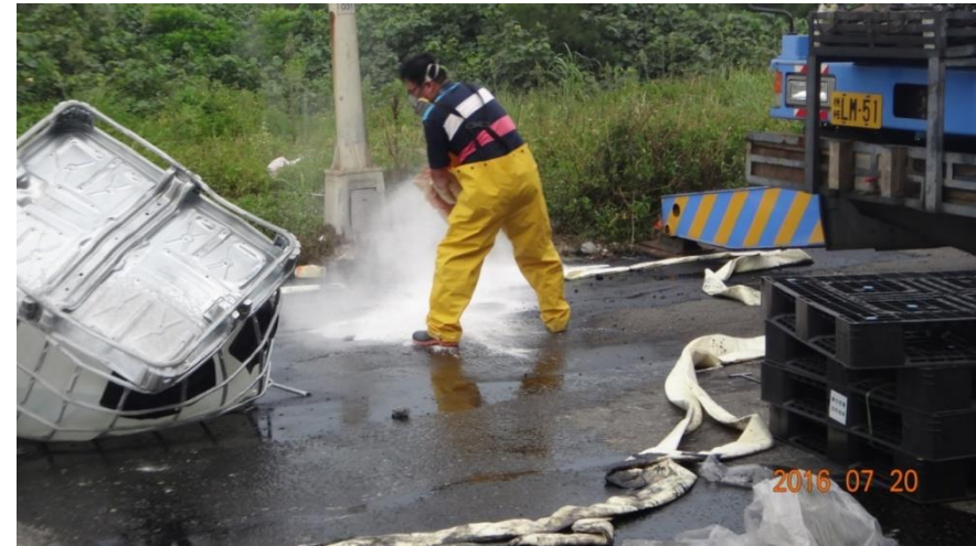
Sprinkle lime on the ground, neutralize sulfuric acid
